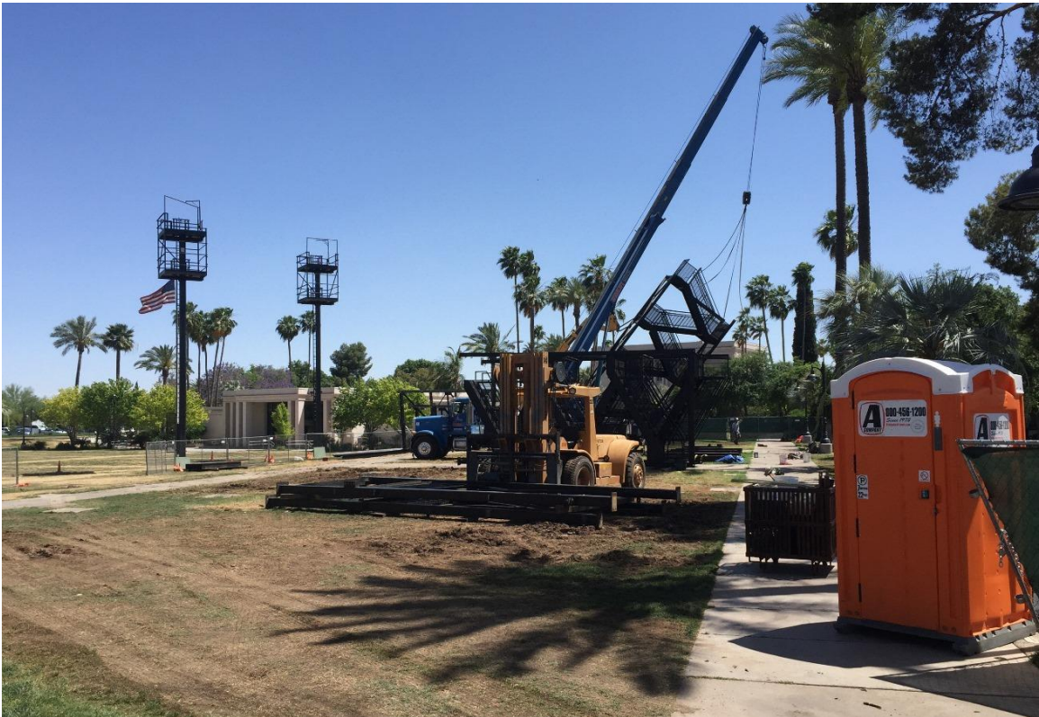
Figure 56: Crane extracting portions of the Easter Pageant Stage – 21 April 2015.
