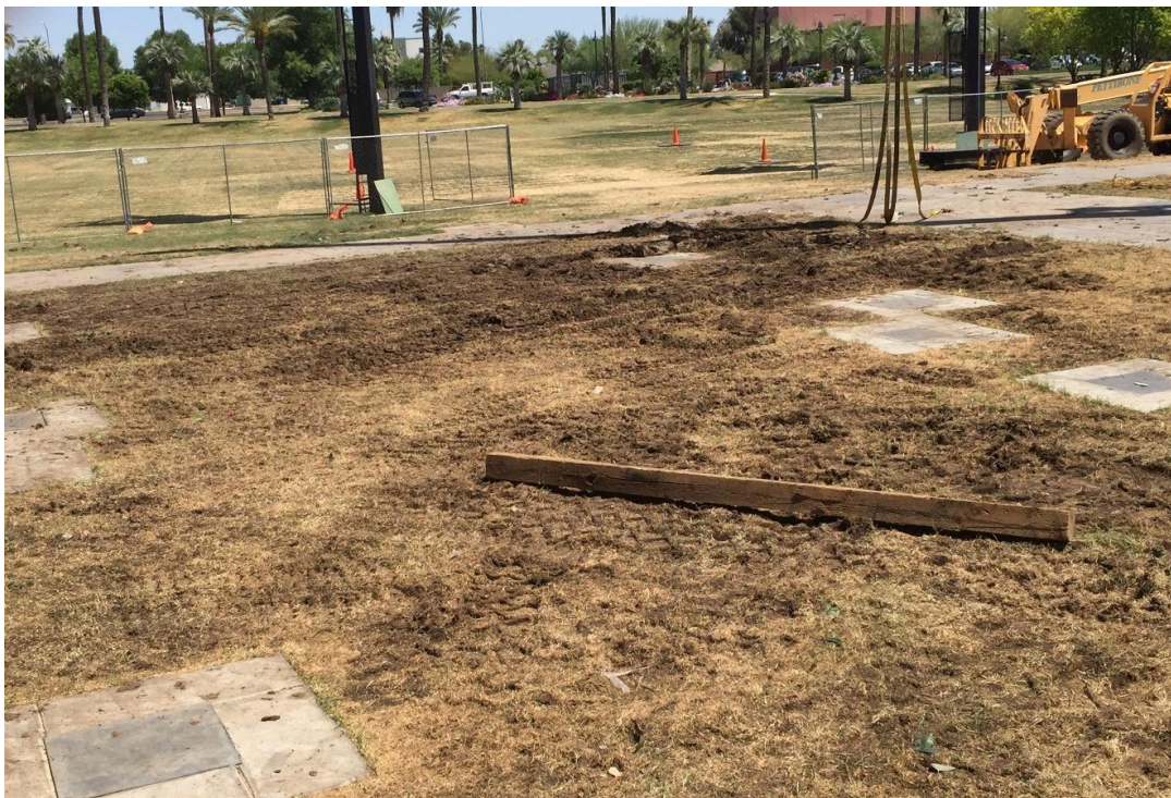
Figure 58: Severe turning damage in the center portion of the Easter Pageant stage area – 21 April 2015.
