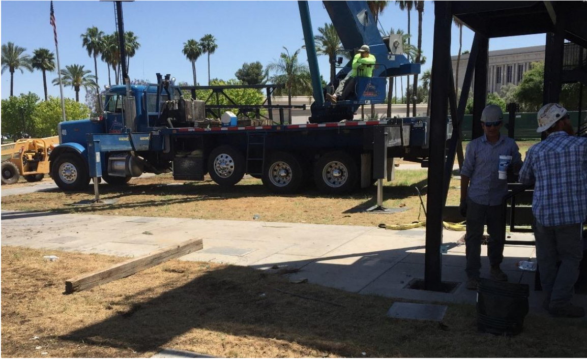
Figure 55: Crane removing the center portion of the Easter Pageant Stage – 21 April 2015.
