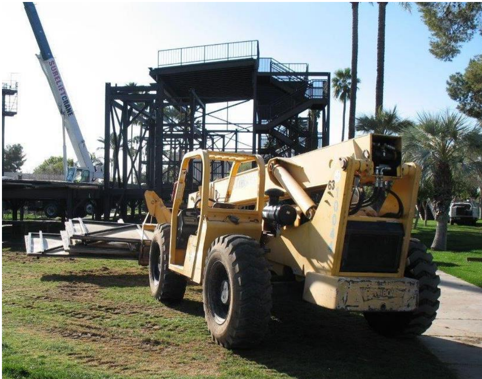
Figure 52: Telehandler in Easter Pageant area during stage construction - 23 February 2015.
