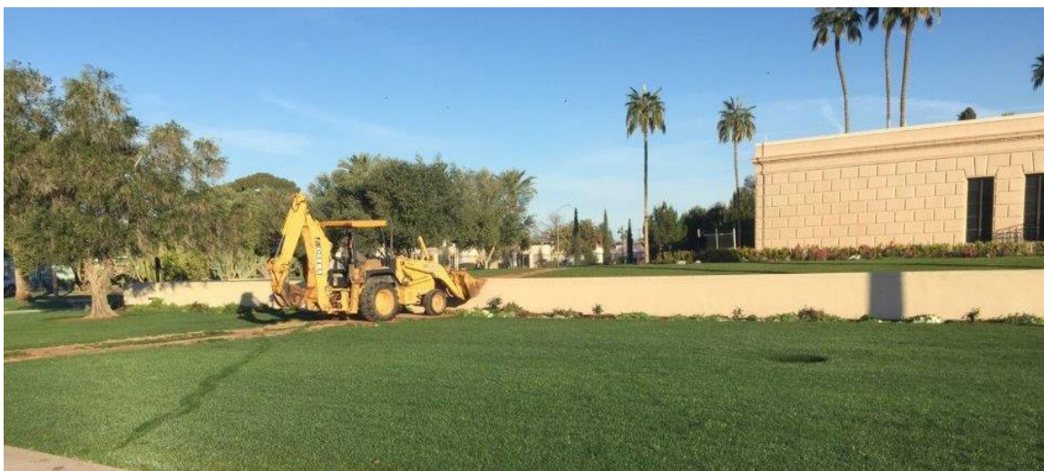
Figure 36: Backhoe on the South Lawn as part of an 8-day construction event during January and February 2015. Notice the turf damage related to the backhoe path.
