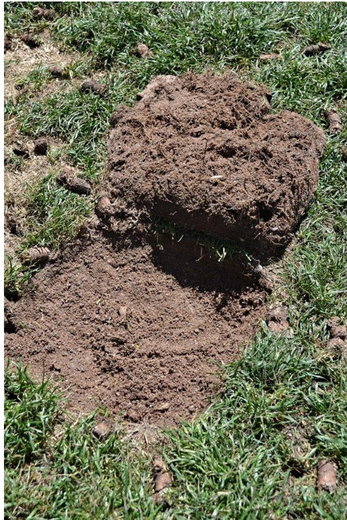
Figure 22: Sod patch on the Northwest lawn rolled back to expose the coarse sand bedding. This picture was captured approximately two months after the sod was laid and demonstrates the shallow rooting depth.
